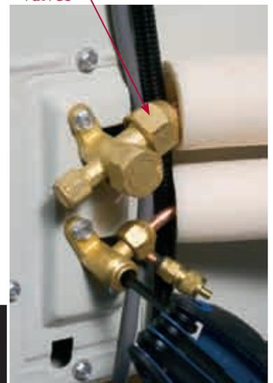
Open the refrigerant gas valves only once you have checked the connections are all made correctly and are tight
