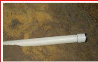
50mm Scour Drain for Cleaning
